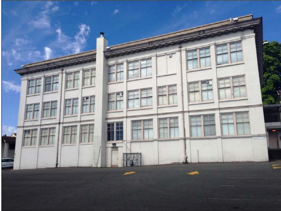
Figure 11. Photo of the east side of the Longfellow Building, facing west. Notice one bank of windows has been covered or removed on the third floor.
