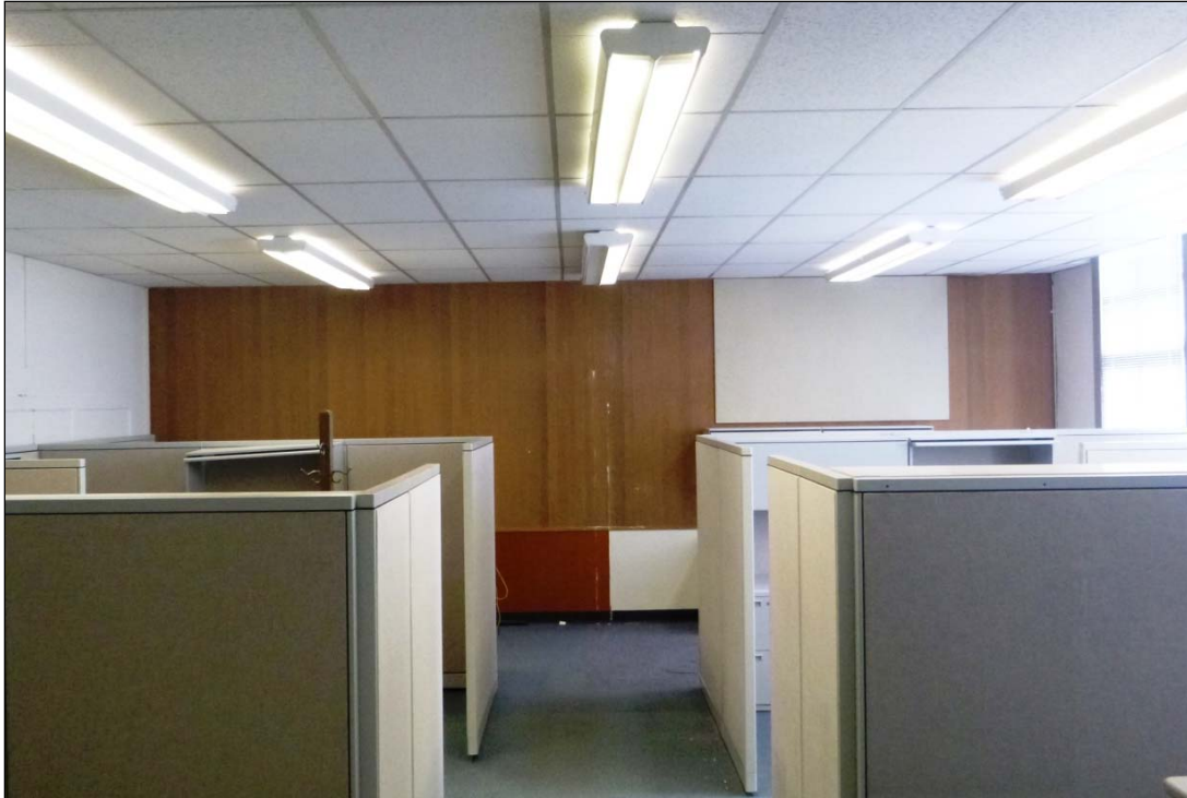
Figure 13. Photo of the interior of the north wall showing vertical wooden slats where windows once were; photo facing north.
