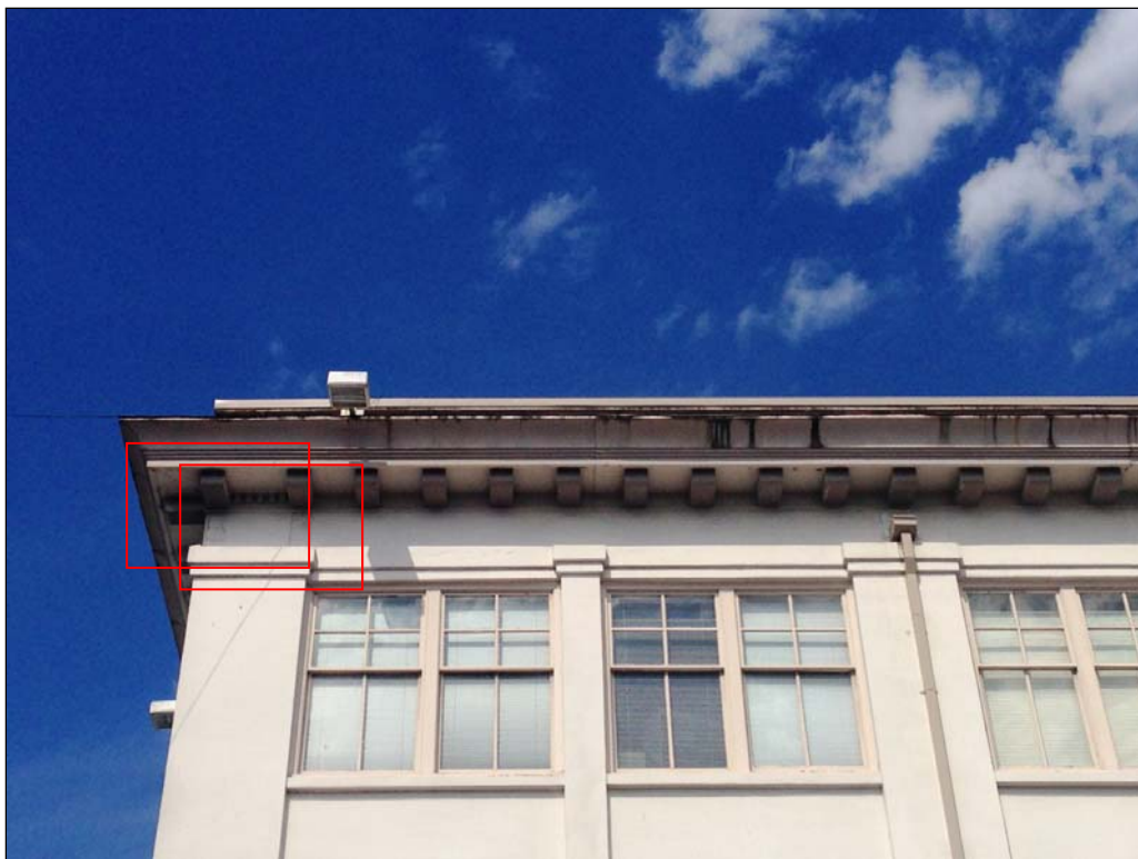
Figure 6. Close up of the entablature with the location of two missing brackets visible (see red box).
